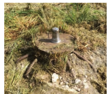
Pershore Bridge, Mortar Spigot base as it can be seen today
