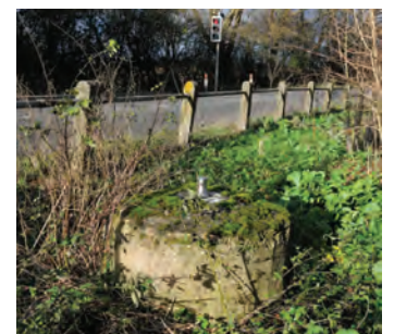
Mortar Spigot site, Eckington Bridge
